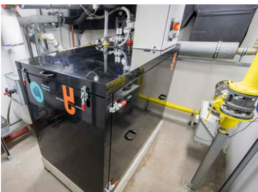
Combined Heat and Power Unit in the Heating Cellar and Local Heat Network © ahnenenkel.com/Silke Reents
